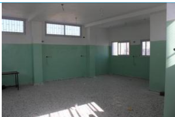
Interior painting works finished
