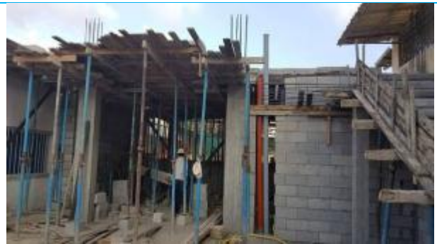
Concrete ceiling and building bricks
