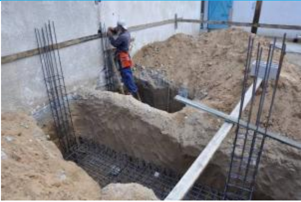
Foundations and column necks
